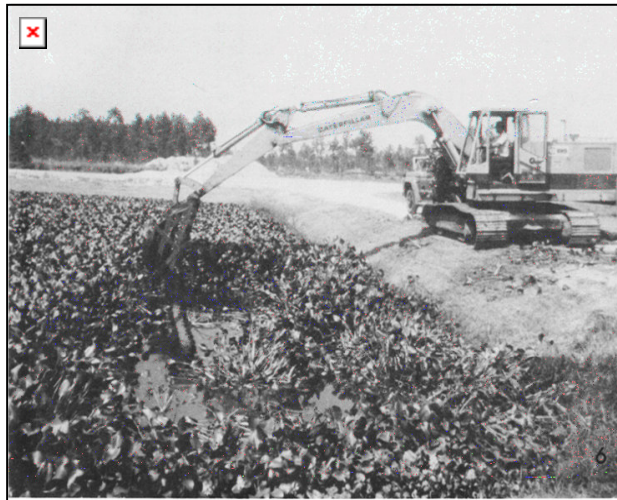
a) Modified bucket attached to a back hoe
