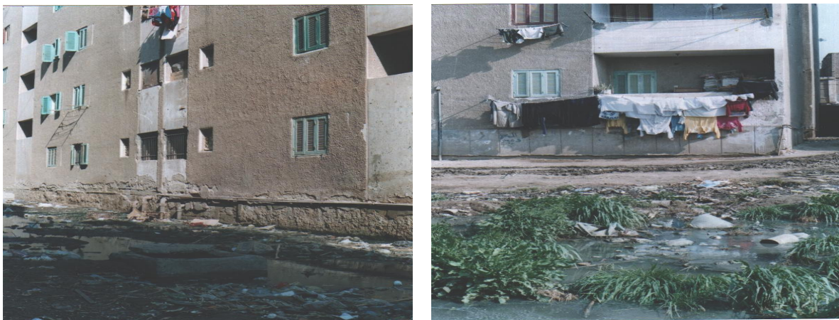
Figure 5 Flooded wastewater in the surrounding areas of septic tank and agriculture land
