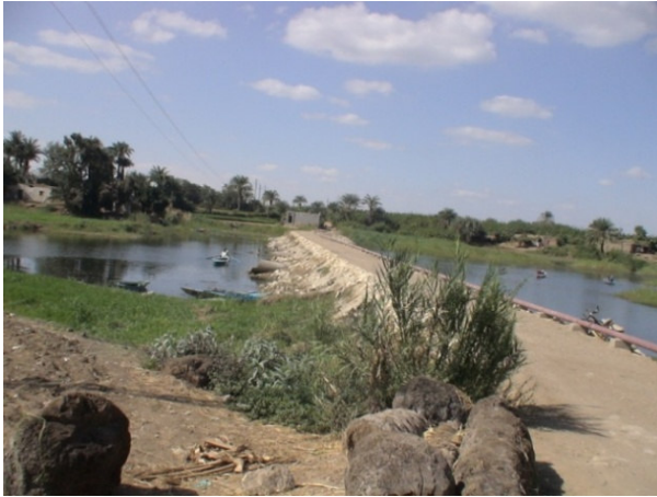
Picture (3) Upstream Roadway
