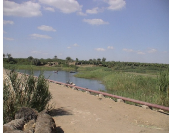
Picture (4) Downstream Roadway
