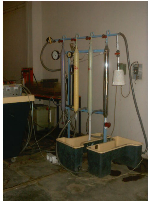
Plate (2): photograph of hydraulic system of water filter
