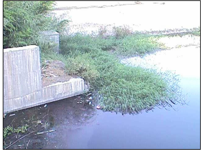
Figure (2) Aquatic Weeds in the Suction Basin
