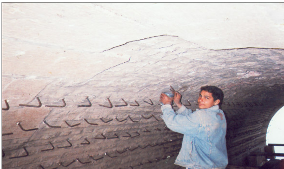
Photo 2 Dowels Planting Process in one of the Arches
