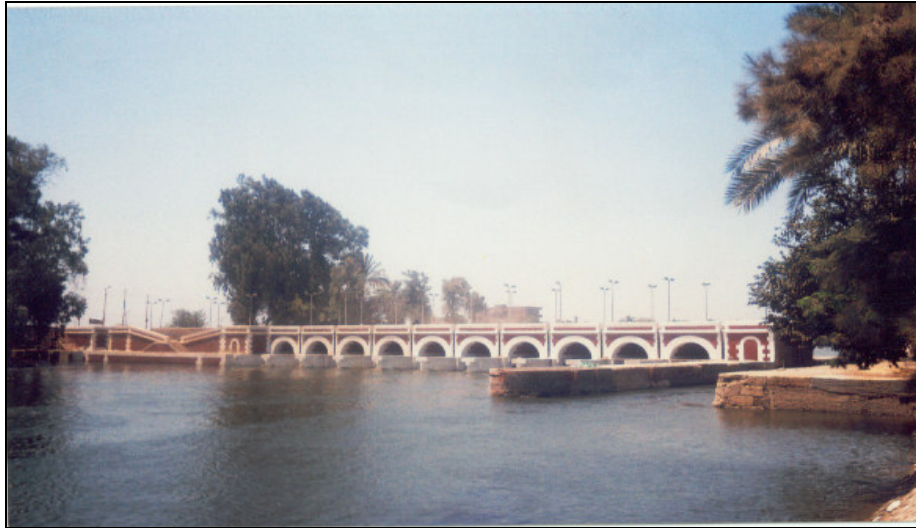
Photo 1 General View for the Barrage
