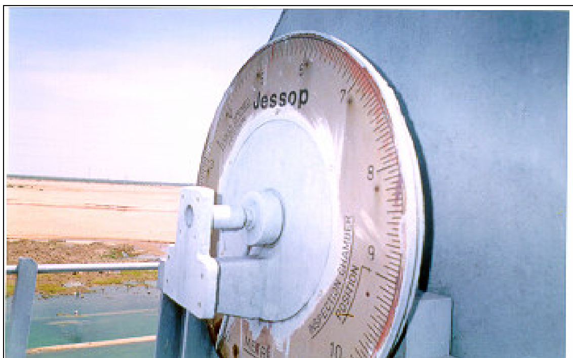
Fig. 9 Gate movement Dial with Encoder mounting device
