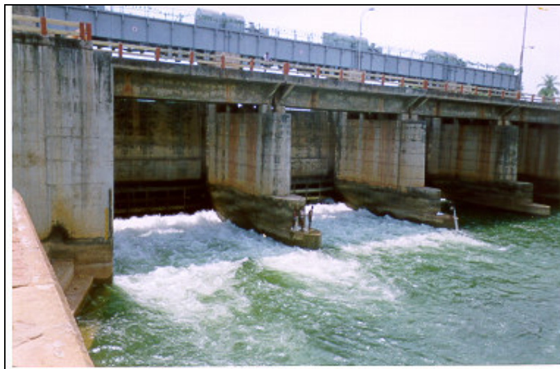
Fig. 8 Barrage Gates in Operation
