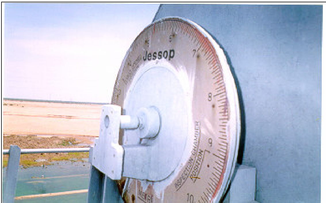
Fig. 9 Gate movement Dial with Encoder mounting device
